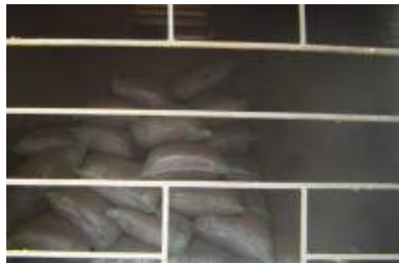
Room in the Bus Stand, being used to store cement bags
