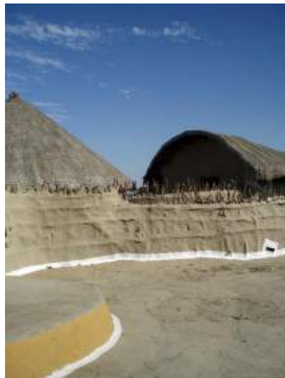
Shaam-e-Sarhad - The design and layout of the resort is based and inspired from the form and structure of the villager's homes in their hamlets, Hodka
