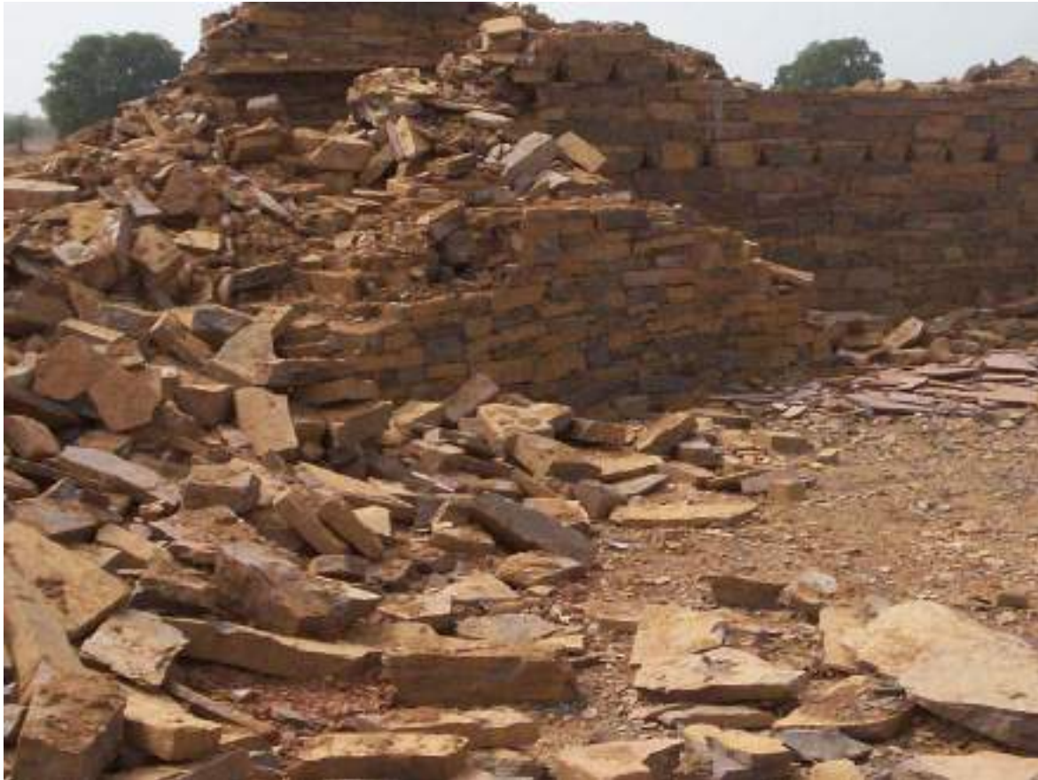
Physical structure of shops brought down as a result of conflict
