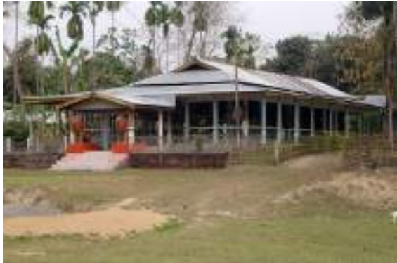
Renovation of the Naamghar, Durgapur
